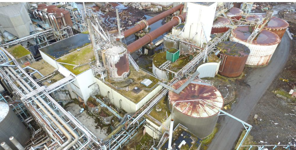
Watson Island prior to commencing clean-up
