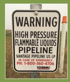
Markers and warning signs are located at frequent intervals along the pipeline ROW. They're found where a pipeline intersects a street, highway, railway or waterway, and at other prominent points along the route. Markers warn that a pipeline is located in the area, identify the product transported in the line, and provide the name of the pipeline operator and a telephone number to call in the event of an emergency.
